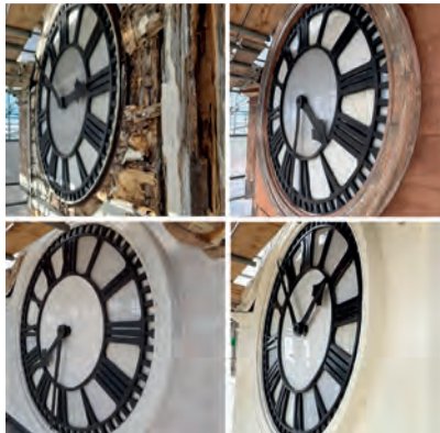
Left: Four stages of the cupola's restoration
